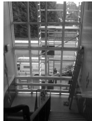
SLE Work in Progress
